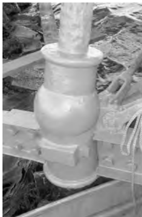
Cast iron coupling at Thomas Point Lighthouse
